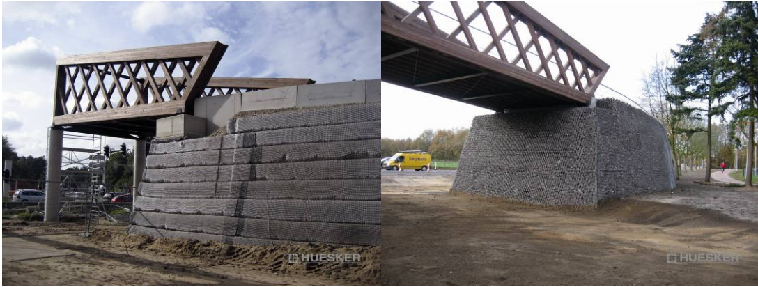
Picture 1. Fortrac ® geogrid reinforced bridge abutment without and with facing (System Muralex ® )
