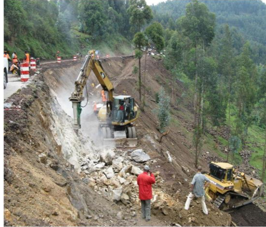
Figure 6: Excavation de la pente existante
