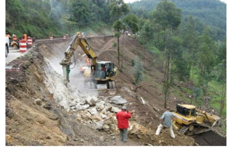
Figure 6. Excavation de la pente existante
