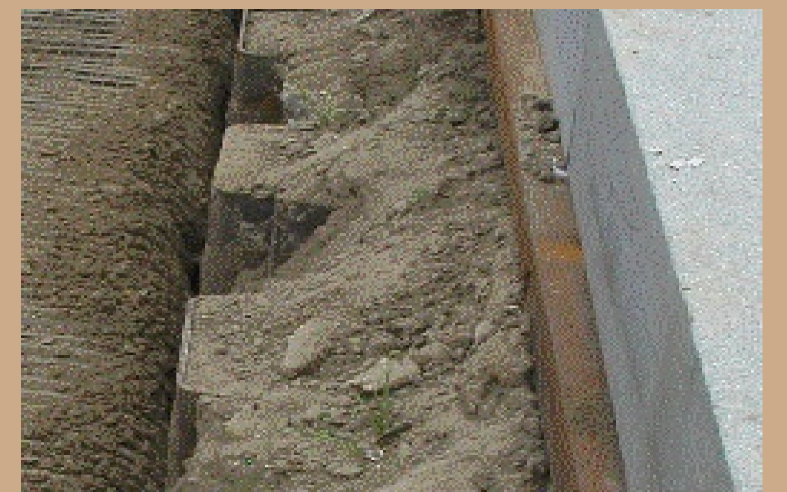
Well tensioned geogrid along the sheet pile wall
