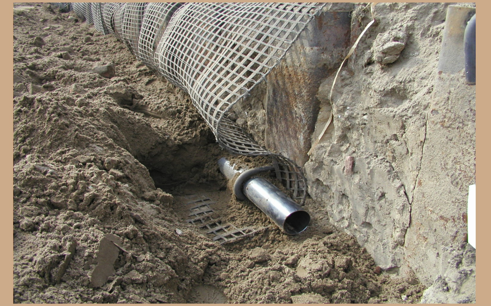
Connection detail between geogrid and sheet pile wall
