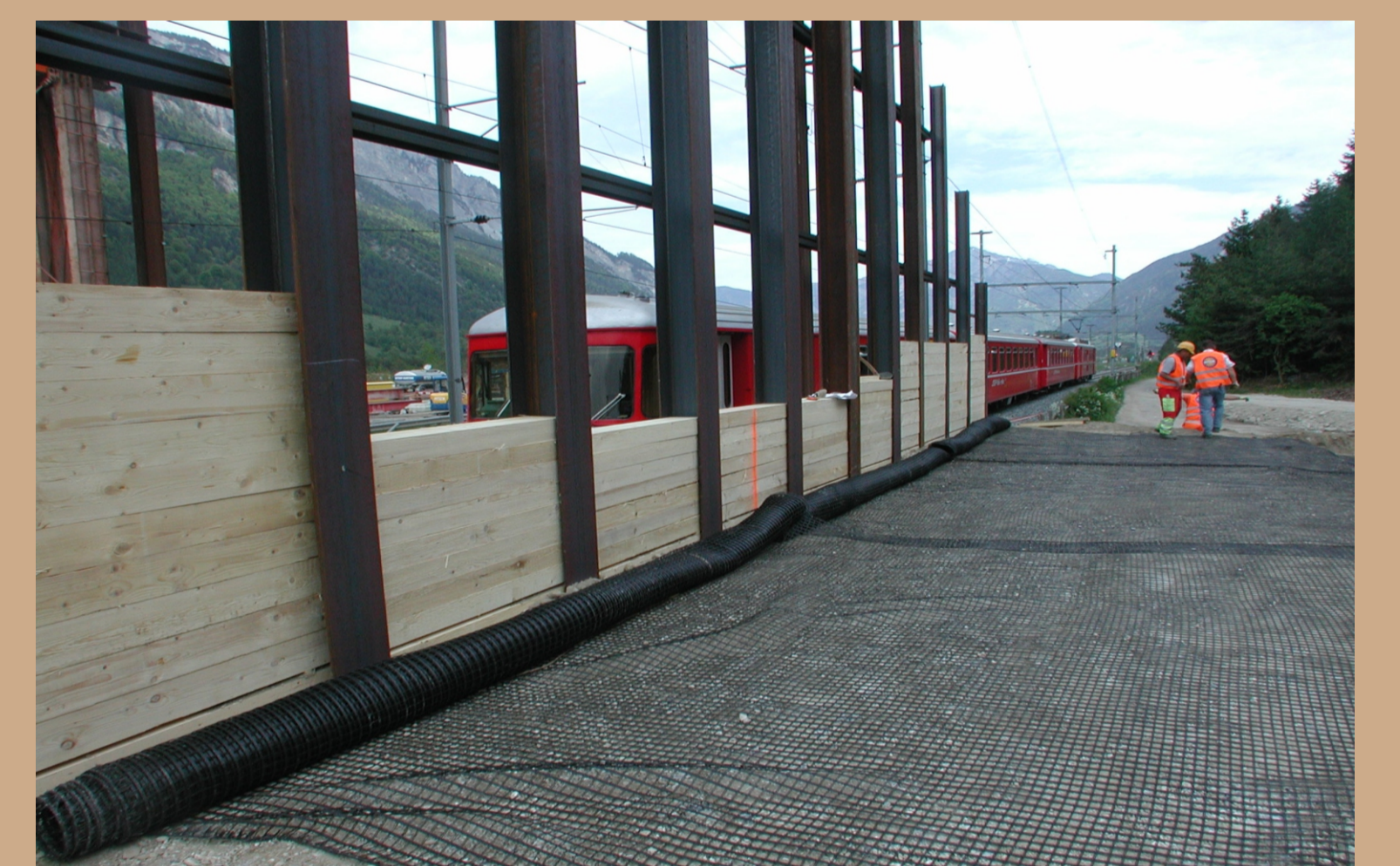
Placing of the geogrids
