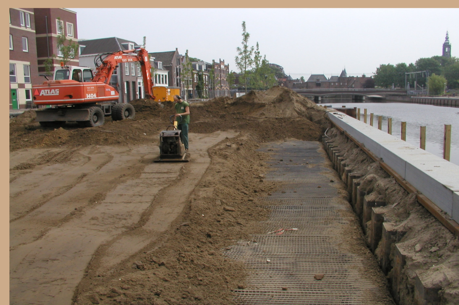
Backfill installation
