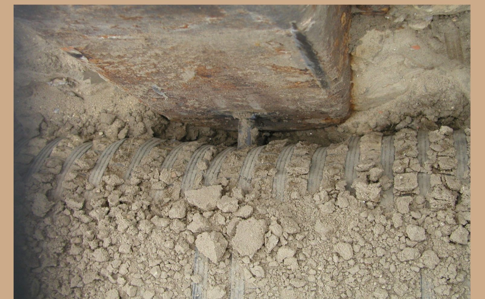
Tensioned geogrid at the connection
