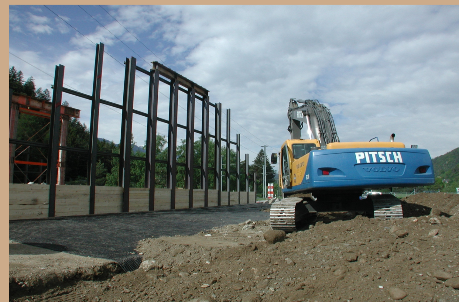
Placing of the geogrids
