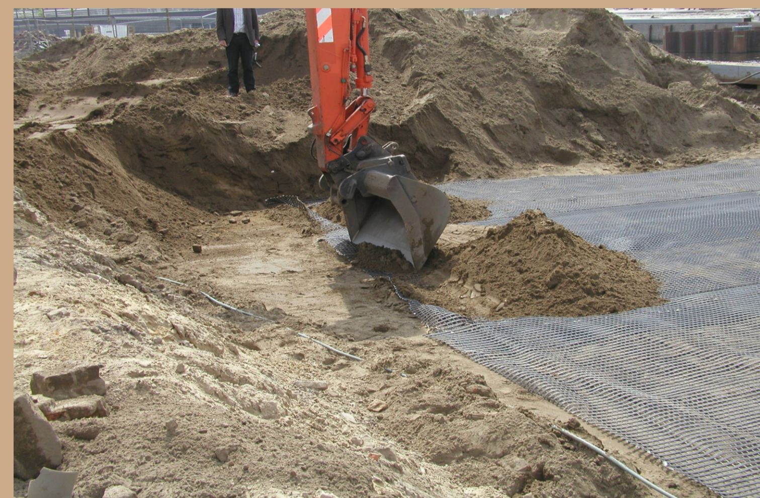
Geogrid prestressing with the excavator shovel
