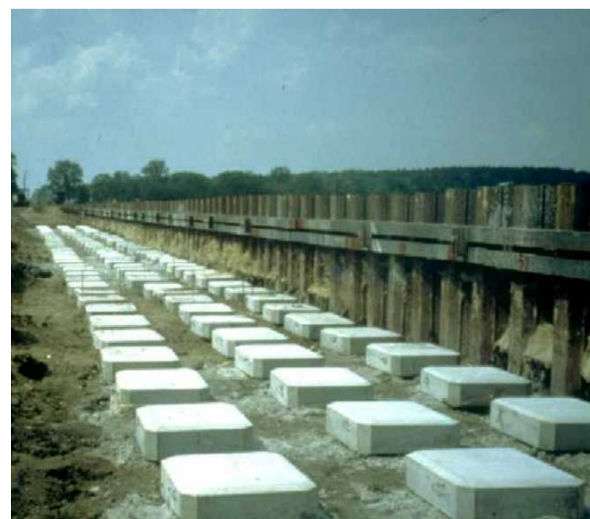
Project Werder-Brandenburg: pile caps before geogrid installation
