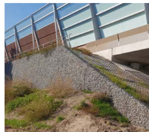
Motorway widening within existing footprint Netherlands | Six-lane widening of (A1/A27) motorway section near Utrecht – Natural sloping motorway embankment rebuilt as steep slope with Fortrac Gabion tie rod system – Erection of top noise barrier made possible by integration of concrete pile supports in system.
