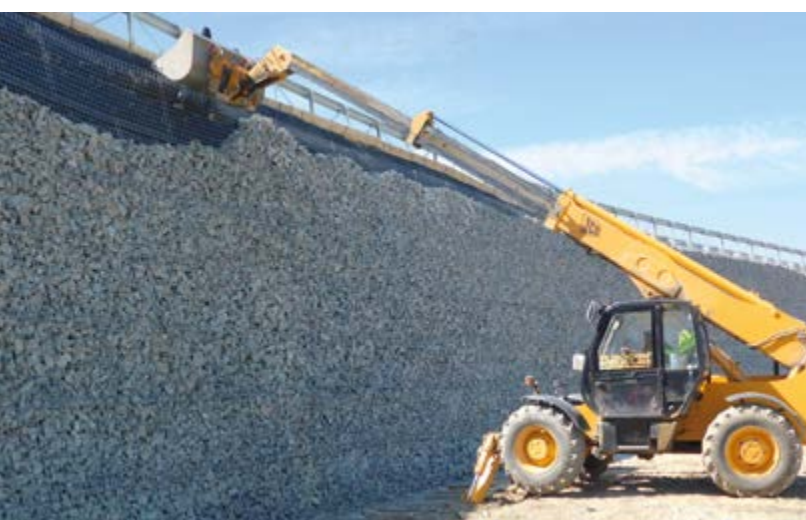
Approach ramp for new bypass motorway Romania | 200 m long, 11 m tall approach ramp (A4 motorway, Constanța-Poiana) – Tie rod system – Special steel mesh aperture size – Rapid progress on site e.g. through simplified filling operation with easy-to-use plant and (140 mm dia.) natural fill material.
