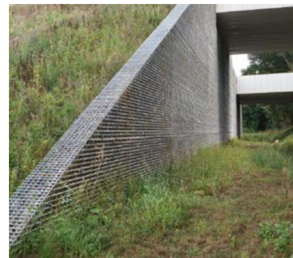
Double bridge abutment for A74 motorway Netherlands | Major project near Venlo, incl. two motorway bridges directly adjacent to each other – Abutment heights 11 m and 9 m – Rapid completion on very soft subsoil – Phased installation after advance surcharging – Tie rod system.
