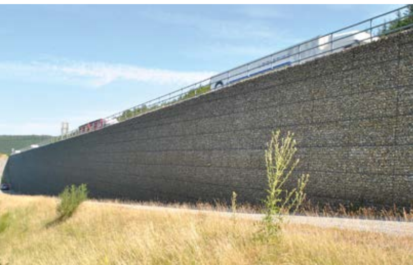
A3 motorway widening, Frankfurt/Main – Würzburg Germany | Embankment widening for new six-lane motorway sections east and west of Haseltalbrücke bridge – Up to 13 m tall full-gabion walls – Self-supporting GRS retaining wall with purely cosmetic gabion facing (passive construction).
