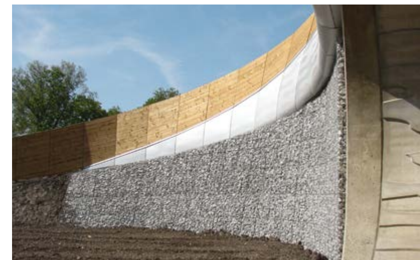
Modern wildlife bridge over A2 motorway Netherlands | Vegetated wildlife bridge over A2 motorway – Curved approach ramp topped by modern architectural feature – Fortrac-reinforced soil system applied in conjunction with half-gabion facing – Height approx. 8 m.
