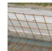
Ungalvanised steel formwork units
