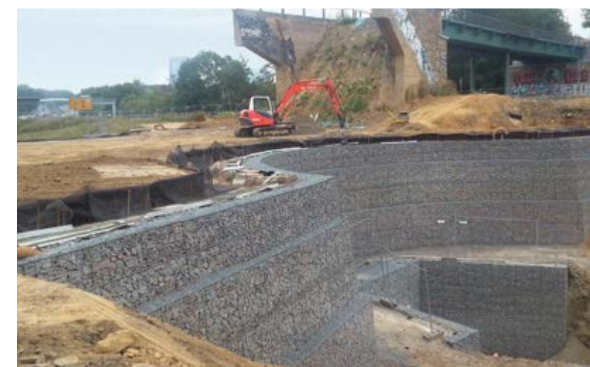
Uncovering of River Schondelle Germany | Sub-project of River Emscher ecological improvement scheme – Earthworks built with integrated lost formwork and full-gabion facing – Solution as replacement for originally planned concrete cantilever wall – Erected in three, 5 m tall vertical sections.
