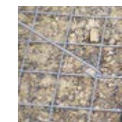
Galvanised steel formwork units
