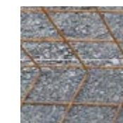
Lost or temporary formwork for passive facing
