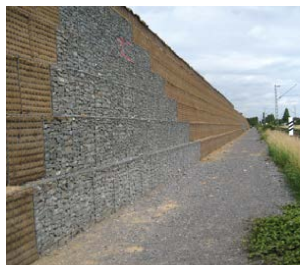
Noise barrier for residential estate in Neuss Germany | Development area by railway and regional road – Combination of full-gabion wall facing track and natural slope facing new housing – Gabions filled with stones, soil and vegetation – 10 m tall with 68° inclination on track side.
